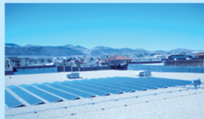
Project: Kohl's department store Megawatts: 0.1 Location: Denver, CO
