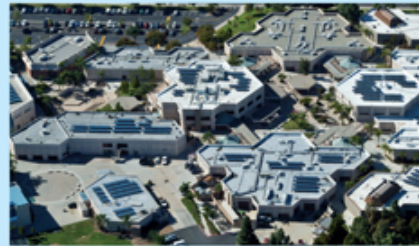
Project: Irvine Unified School District Megawatts: 0.2 Location: Irvine, CA
