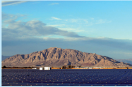
Project: Mt. Signal Megawatts: 265.7 Location: Calexico, CA
